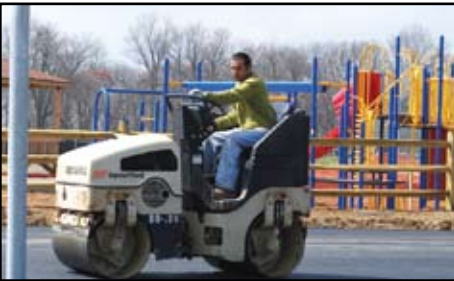
Beginning the paving process for the basketball court!
